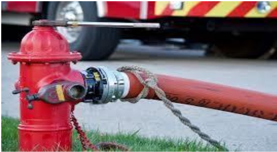
FIRE HYDRANT WITH HOSE CONNECTED
